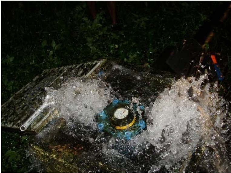
Repairing the 150mm meter of the line from the Sarakata Reservoir
